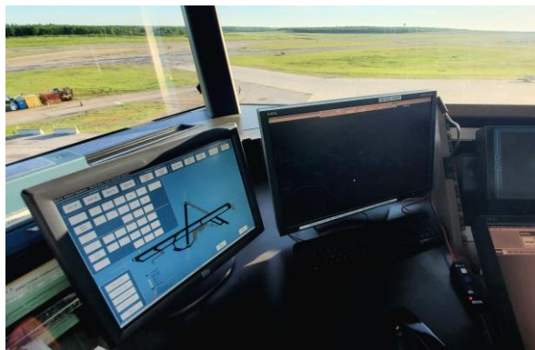
◀ Airport Lighting Control Systems, ARCAL, and Computers Replaced
