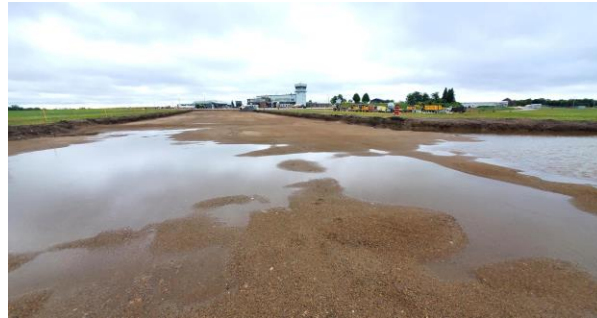
◀ Hotel Taxiway Replacement
