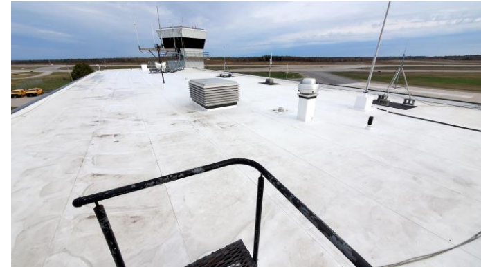
▲ Administration Building Roof Membrane Replacement
