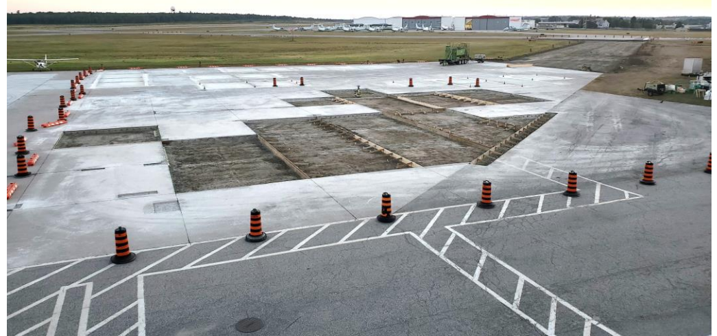
▲ Apron II Selective Panel Replacement and Golf Taxiway Complete Replacement
